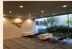
Introduction and renovation of LED lighting (TK Flats Shibuya)
