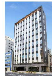
The Nihonbashi Bakurocho 1-chome Development Project ( Daiwa Nihonbashi Bakurocho Building )
