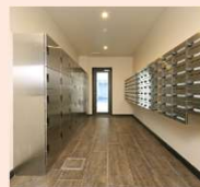
Installation of Delivery box (PREGIO Namba)
