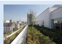
Installation of rooftop garden (Daiwa Azabu Terrace)
