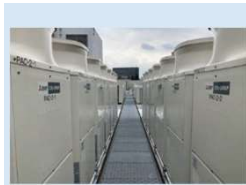
Upgrading of air-conditioning equipment (Daiwa Ginza)
